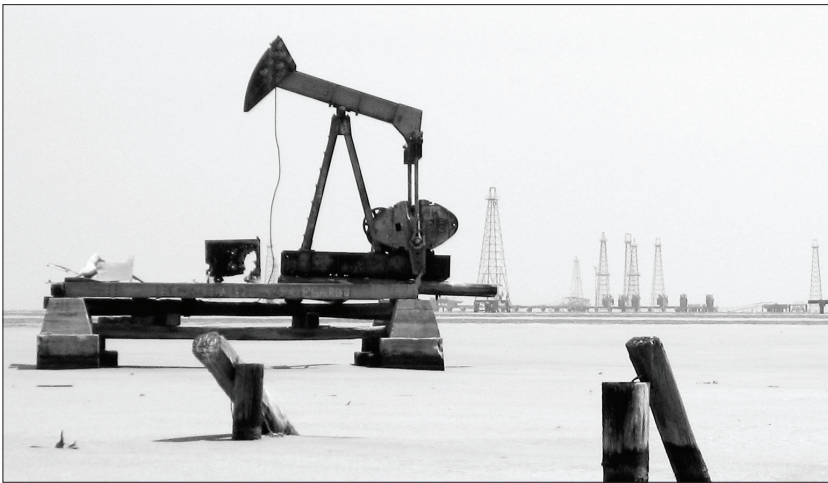
Oil derricks on Lake Maracaibo—duckweed covers the lake's surface
